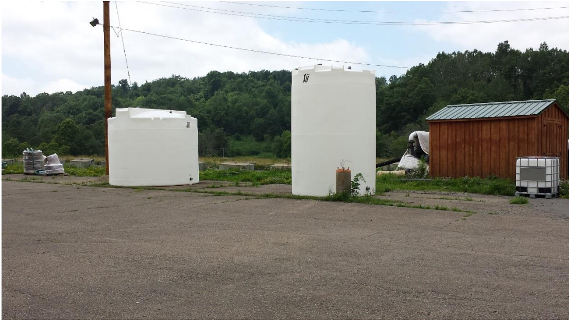
Figure 7: Storage tanks for process byproducts.
