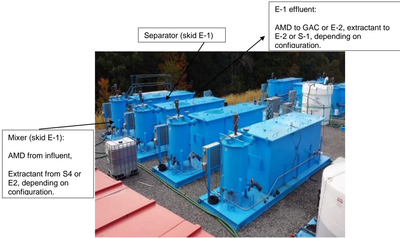
Figure 3: Extraction skids, showing mixer tank and separator.
