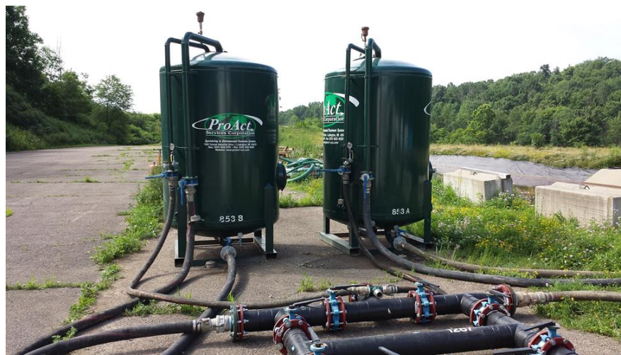
Figure 4: Granular Activated Carbon (GAC) beds used to polish effluent water. Beds were operated in series.
