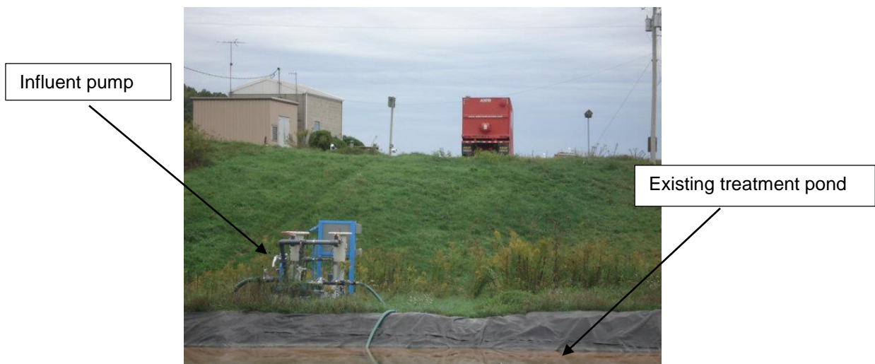
Figure 2: Inlet pump for AMD from outfall of existing treatment pond.
