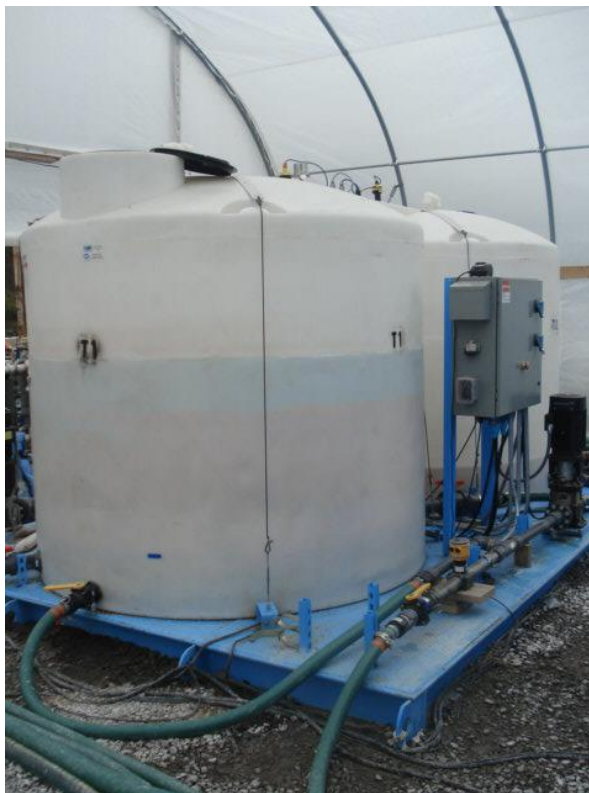
Figure 8: Polished AMD tank (T1, left), and extractant overflow tank (T2, right).
